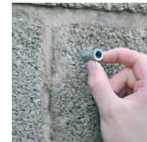
C. Position fixture, tighten bolt into shield
